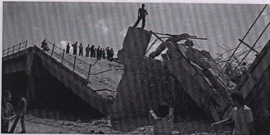
Bridges are regularly targeted by Israel because their destruction harms the economy
